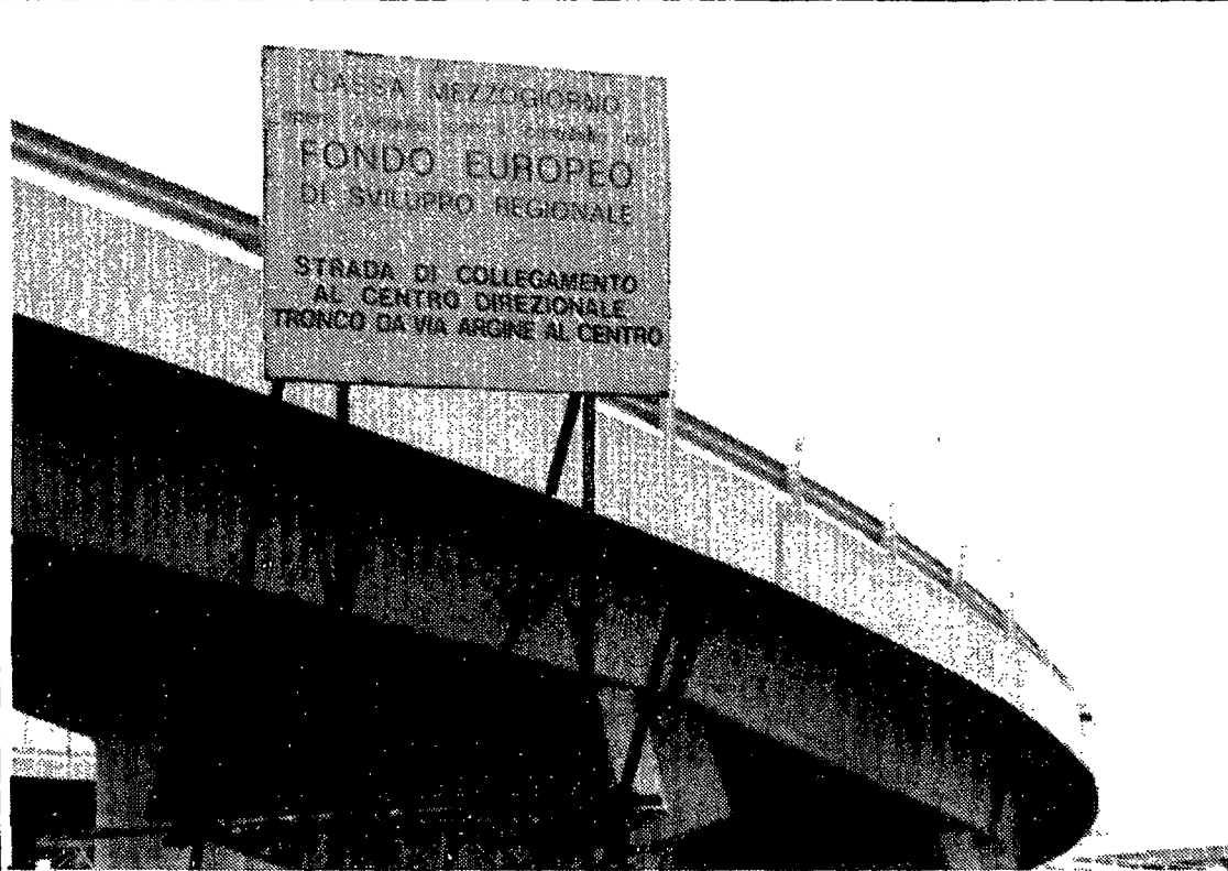
Access road to Naples (Italy)
